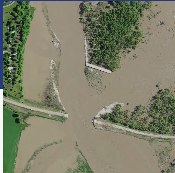
Displaced bridge in USGS/FEMA flooding imagery
